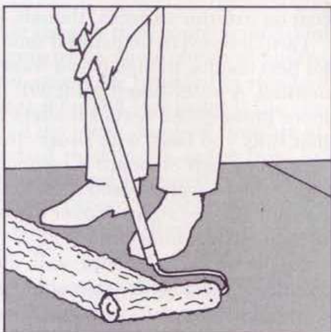
2. Apply a hard-setting casein glue along joints, using a roller.
